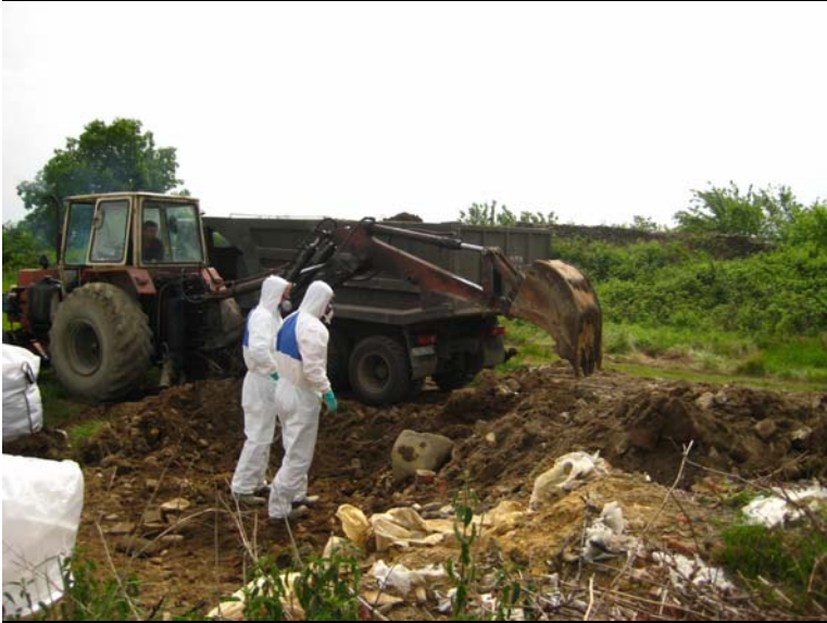
Picture 8.9 Excavation of the contaminated media
