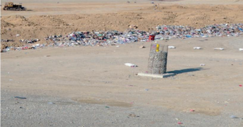
**Photo 6.2.2.1. Part of methane collection system mounted at the Tbilisi new landfill**
