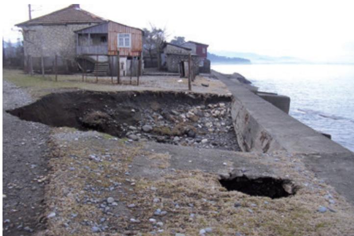
**Photo 6.1.3.1. The funnel-form cavity washed out by the wave behind the wall**
