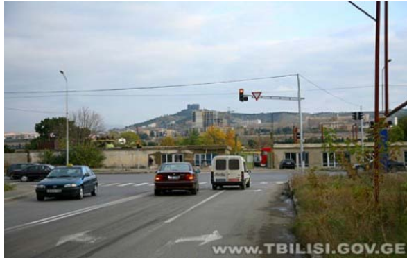
Picture 2: A new traffic light system on the crossing point of Beliashvili and Chachava streets. Source: www.tbilisi.gov.ge
