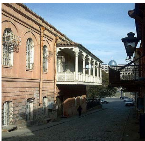
Picture 5: Old building in the central historical part of Tbilisi
