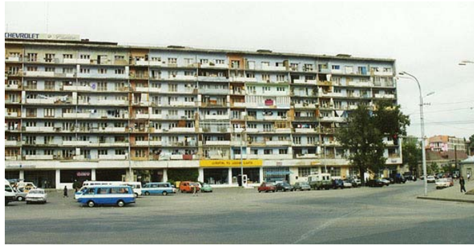
Picture 6: Soviet era multi-apartment building block
