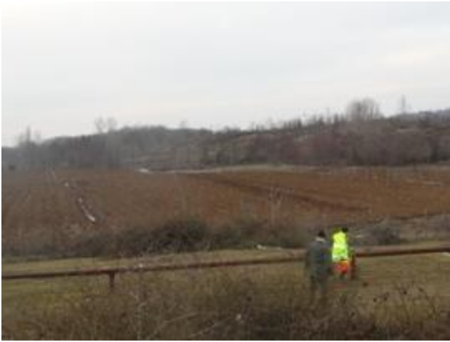
Stripped Pipe across the Agricultural Lands
