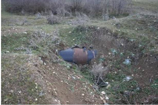
Exposed and Stripped Pipe Sections
