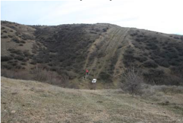
Pipeline ROW Going Uphill
