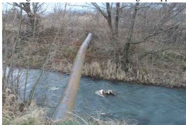
Corroded Pipeline over the Channel Crossings
