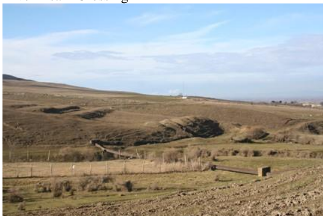
Stripped Pipe across the Agricultural Lands
