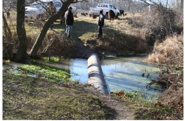
Exposed Pipeline Sections in the Water across the Channel Crossings
