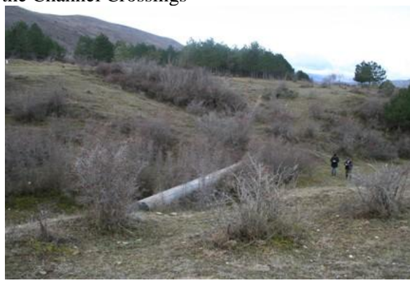
Stripped Pipeline Overgrown with small Trees
