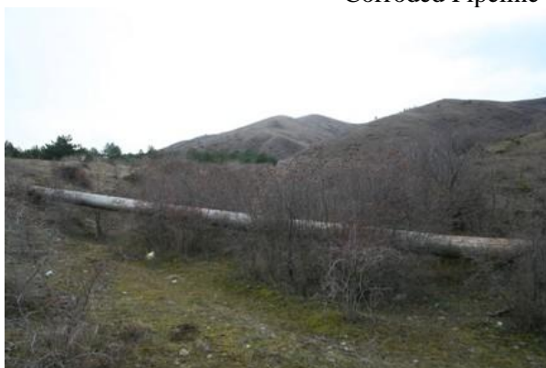
Stripped Pipeline Overgrown with small Trees
