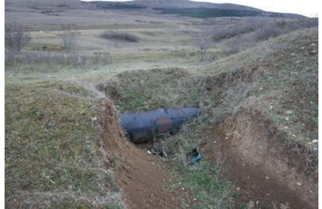
Exposed and Stripped Pipe Sections
