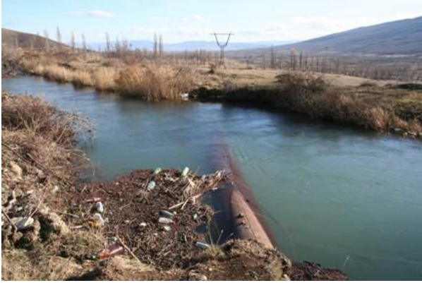
Exposed Pipeline Sections in the Water across the Channel Crossings
