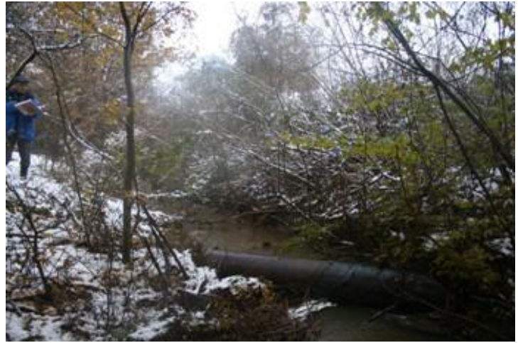
Stripped Pipe Inside the River Western Tortla
