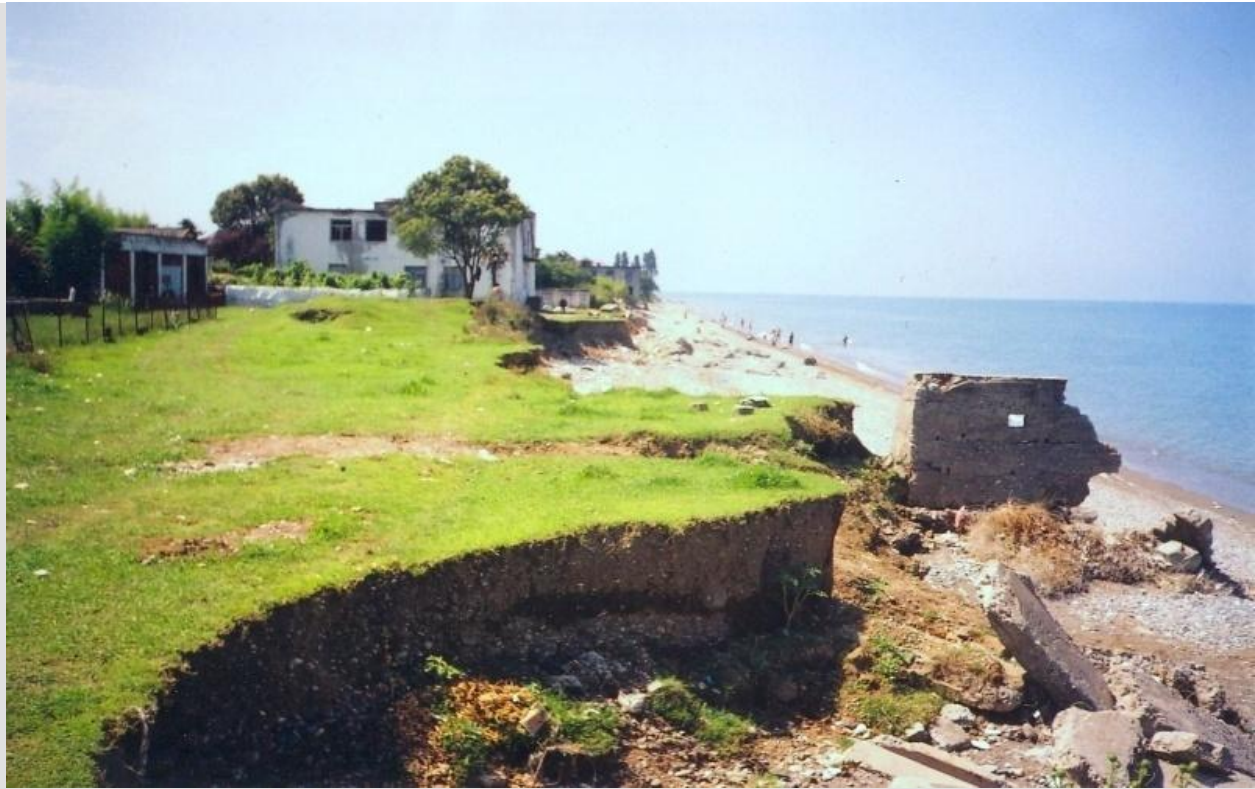
Photo 1. Water erosion process in Adlia segment of the Black Sea coastal zone
