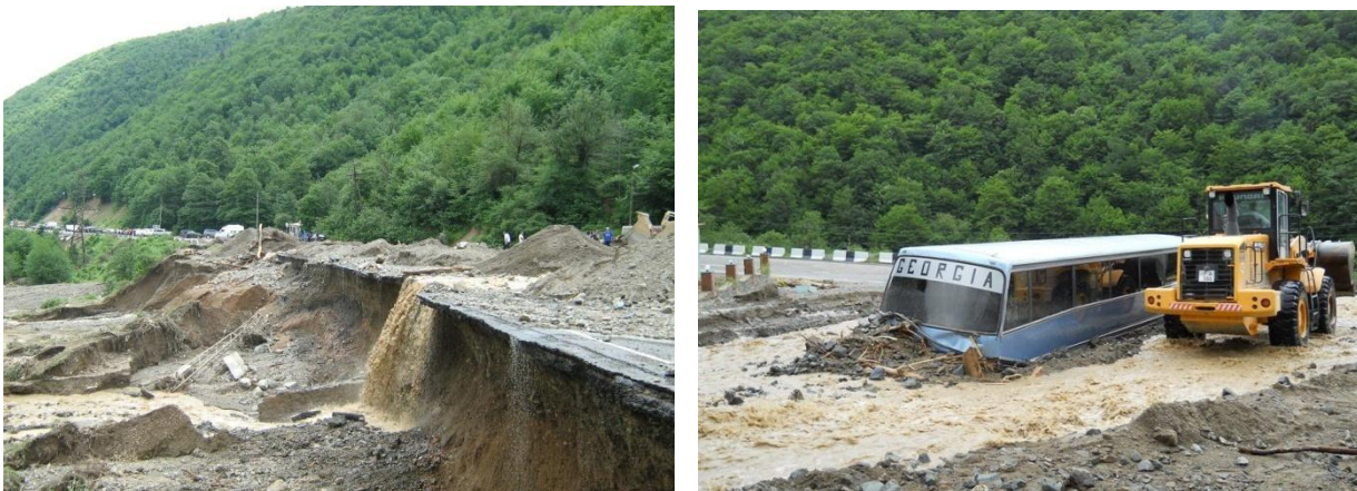
Photo 2. Most recent extreme geological event. 18 June 2011. More than 100 mm rain during two hours were observed on 18 June 2011 at the Rikoti Pass. As a result 6 persons were died, highway infrastructure was destroyed in this segment and more than 1000 housing estates were flooded and damaged by mud stream.
