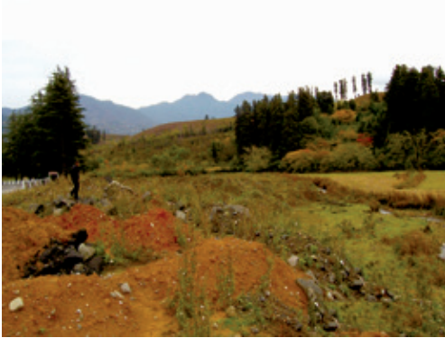
Photo 6.1.1.4. The agricultural land (8 ha) damaged with barren rock
